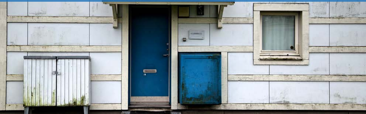
Refurbishment of 493 town houses in Albertslund, Denmark SEK 610 M
