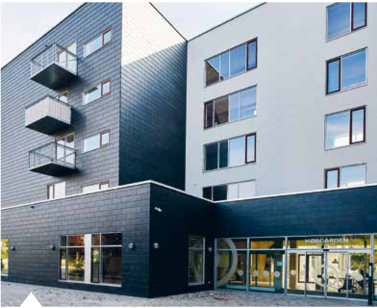
NCC is energy refurbishing the Hørgården residential home for the elderly, outside Copenhagen. When everything is completed, the residents will have modern, healthy, spacious and bright housing units. Read more on p. 25.
