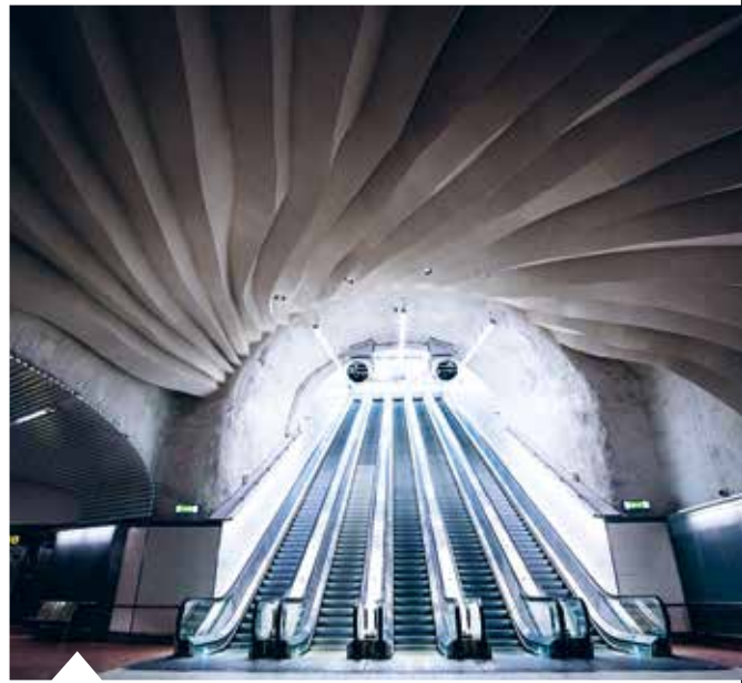
In 2017, NCC completed the assignment to construct the Norrström Tunnel and coordinate the completion of Stockholm City, the new commuter train station. Read more on p. 23.
