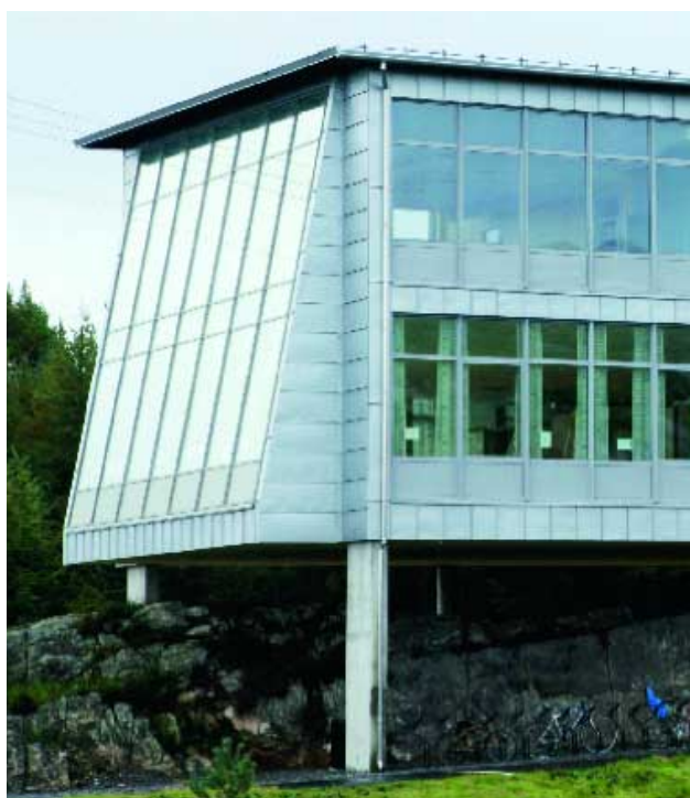
The Sund Department of Sotra Senior High School outside Bergen, Norway, was designed and built in harmony with nature. Rooms with large glass sections admit an abundance of light and provide a sensation of close contact with the natural surroundings. The interiors are also hallmarked by their open-landscape layout. The school was designed by Fortunen, a Norwegian architectural firm. Photo: Henrik Ottosson
