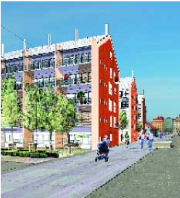
In Sundsvall, central Sweden, NCC is constructing Sweden's first five-story building entirely in wood. It is a unique project involving the use of new production technology. The floors and solid wood wall units are prefabricated. The project also marks the first time that residential apartments have been built in Sundsvall since 1990. White arkitekter performed the design work. 3D illustration: White arkitekter
