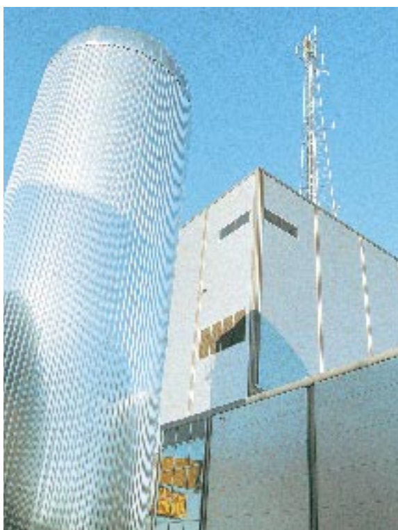
In Märsta, north of Stockholm, the Civil Engineering and the Building business areas are jointly constructing a combined heating power plant based on bio fuels.
