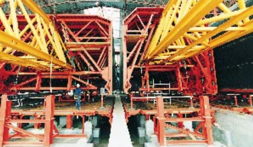
The tunnel segments for the Öresund Link are built under controlled climatic conditions in the specially constructed plant at Copenhagen's Northern Harbor.
