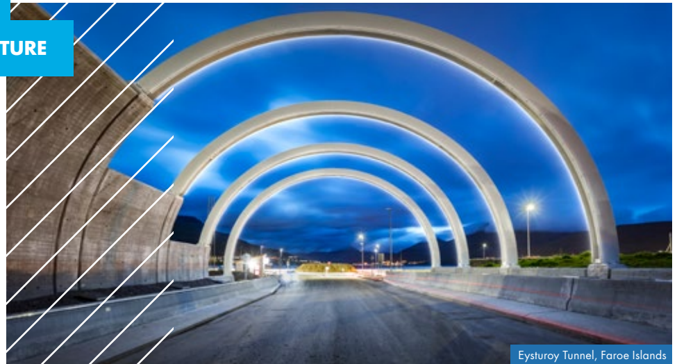
Eysturoy Tunnel, Faroe Islands
