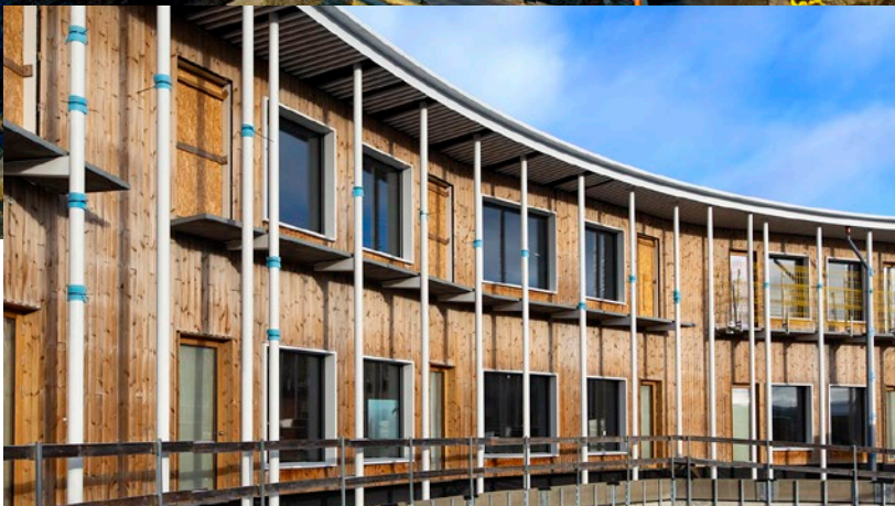
The façades have been installed, and the silver Kalzip roof is taking shape and will be completed in spring 2024.
