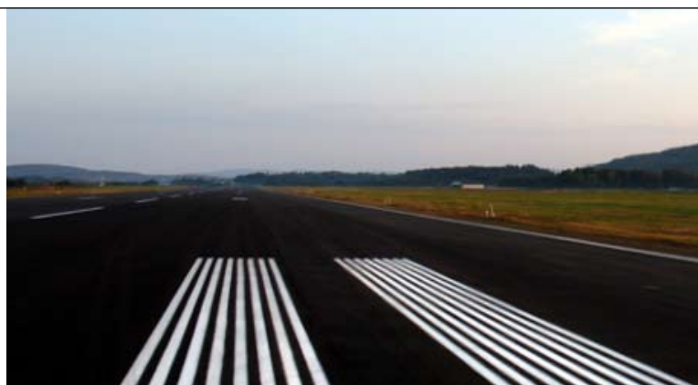
Landing strip at Kramfors/Sollefteå Airport, Sweden.
