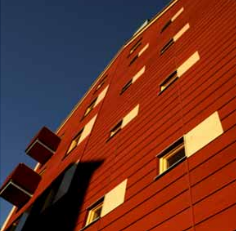
At the Inre Hamnen in Sundsvall, NCC is constructing Sweden's largest wooden residential building to date. The five-floor building, with a total of 94 apartments, is based on a unique design featuring a solid-wood framework and completely wooden-clad façades.
