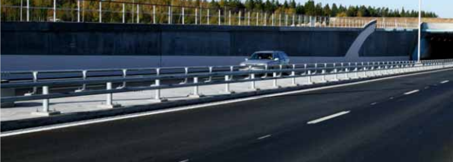
Expressway 26 at Skultorp, in Skaraborg. NCC Roads' assignment included asphalt paving of one of the sections of this project.
