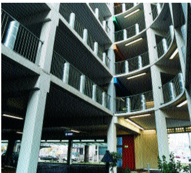
The Koffen parking building at Stena Line's Denmark Terminal in Gothenburg is an NCC-constructed modern parking facility that resolves the parking requirements of the client, Göteborgs Stads Parkerings AB. Well-conceived logistics facilitate traffic flows to and from the building, while a space-efficient layout enabling more cars to park in the limited floor area reduced the construction cost for the customer.
